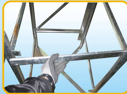
7. Put the bar on back door
